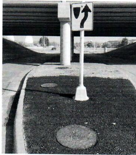
DUROCOM handhole installed near traffic lights.
